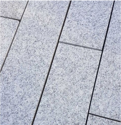
Small Concrete Unit Paving - Plaza Entrance • Flame Exfoliated • 200 x 150 x 40mm
