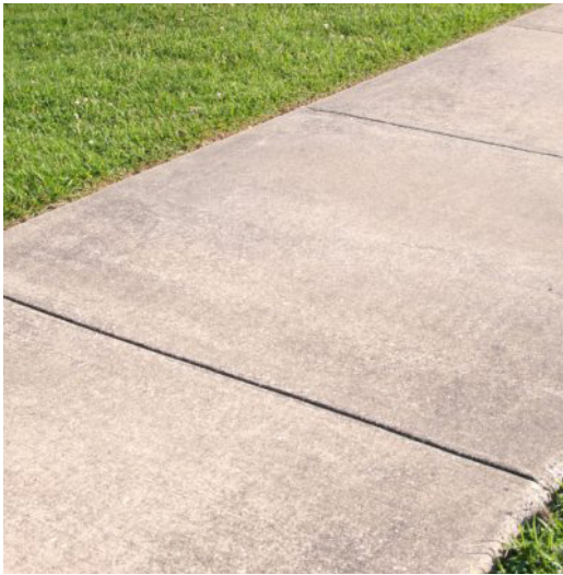
In-situ Concrete Paving (with nature verge) - Streetscape • Natural grey • Broom finish
