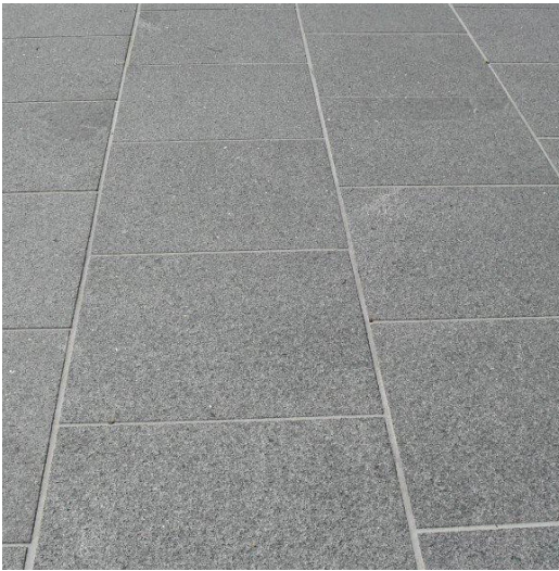
Concrete Unit Paving - Lobby Entries • Flame Exfoliated • 300 x 150 x 40mm
